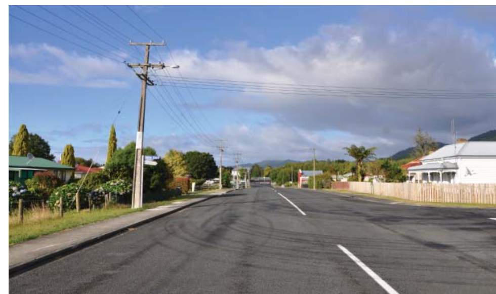
Photo 23. Pedestrian facilities are limited throughout the town
