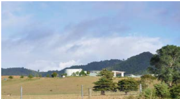
Some of the Waikato-Tainui College building on the hill
