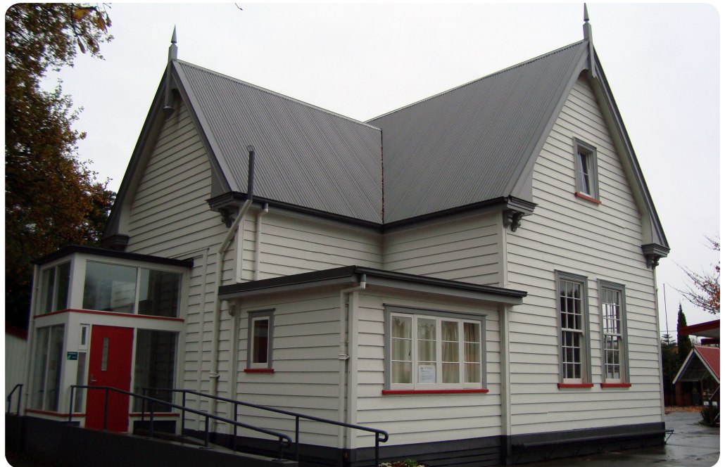
↘ Figure 1. Tamahere School Original Building
