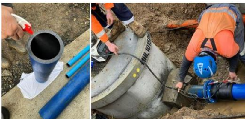
Dominio Road Extension – disinfection solution preparation and handling materials
