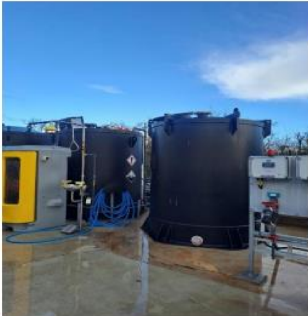
Caustic tank work in progress
