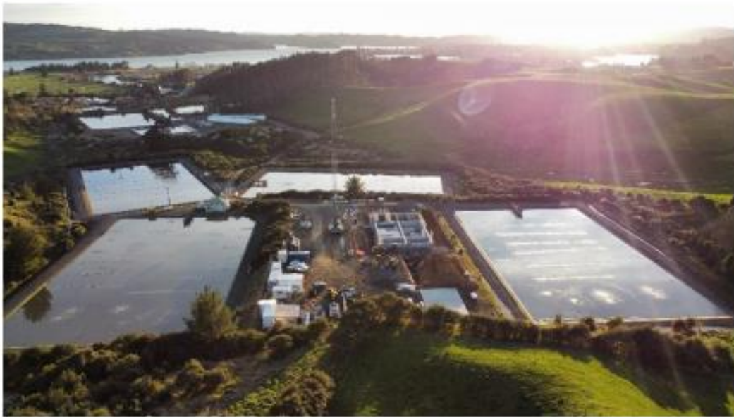
Raglan WWTP MBR Upgrade- The reactor tank and building foundation.
