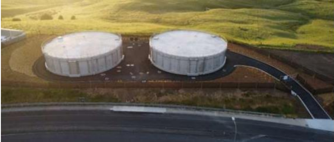
Te Kauwhata Reservoirs - Fully operational
