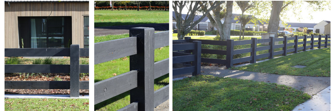
■ ■ RURAL BOUNDARY TREATMENT EXAMPLE - 1.3M POST AND RAIL FENCING
