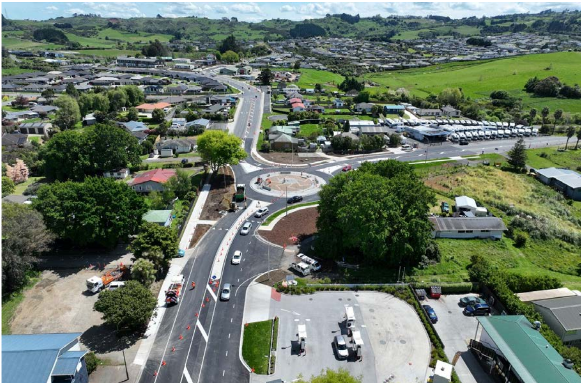
Roundabout site looking north
