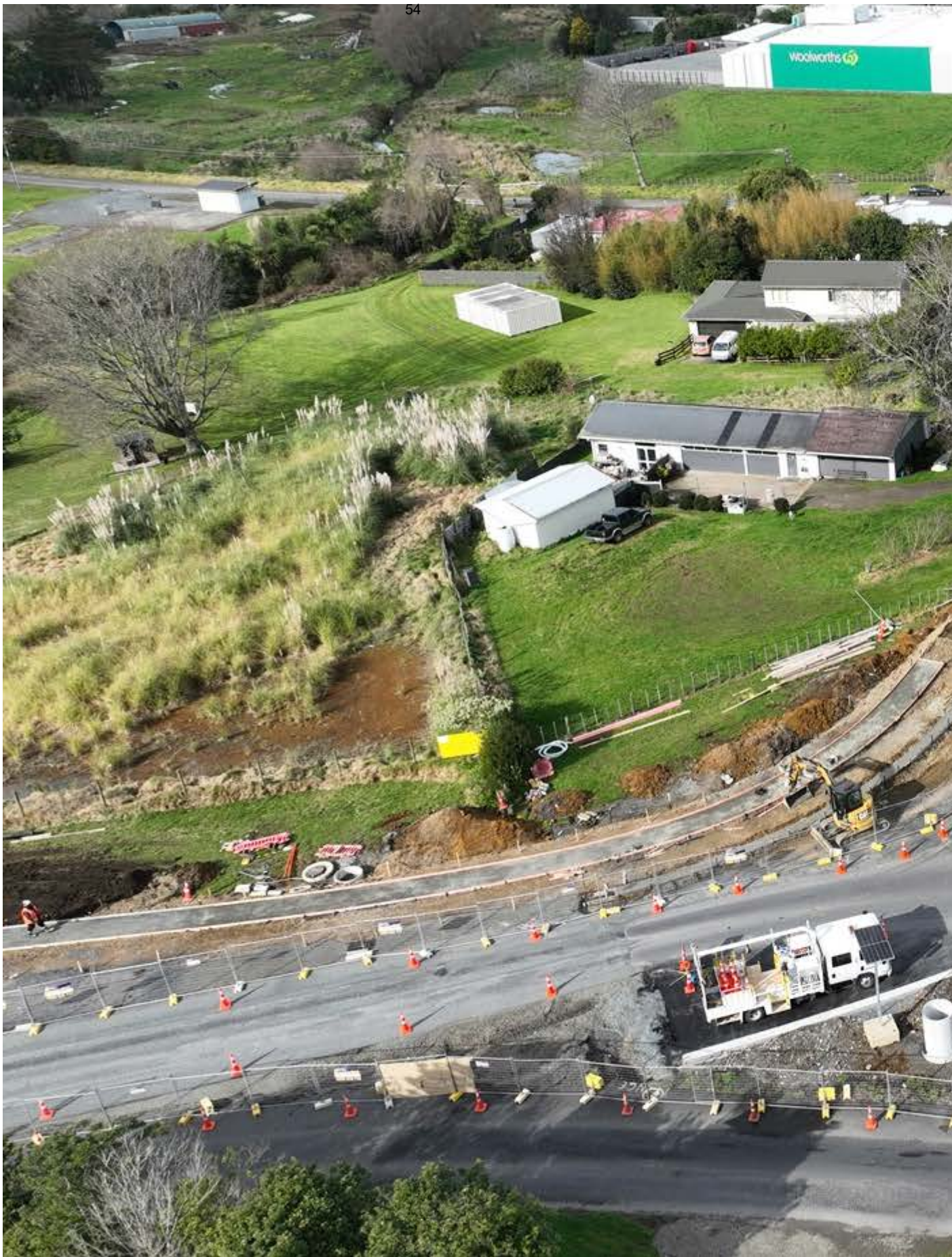
Roundabout site looking south
