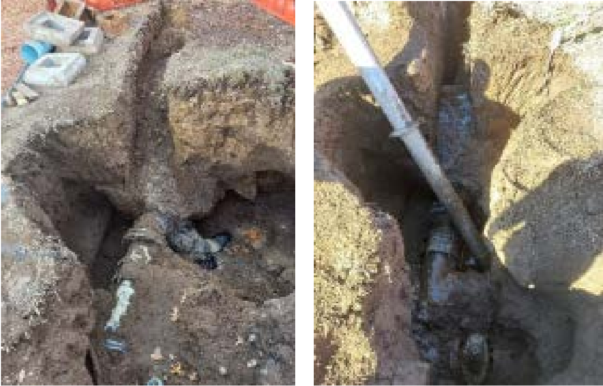
Leak repair works
