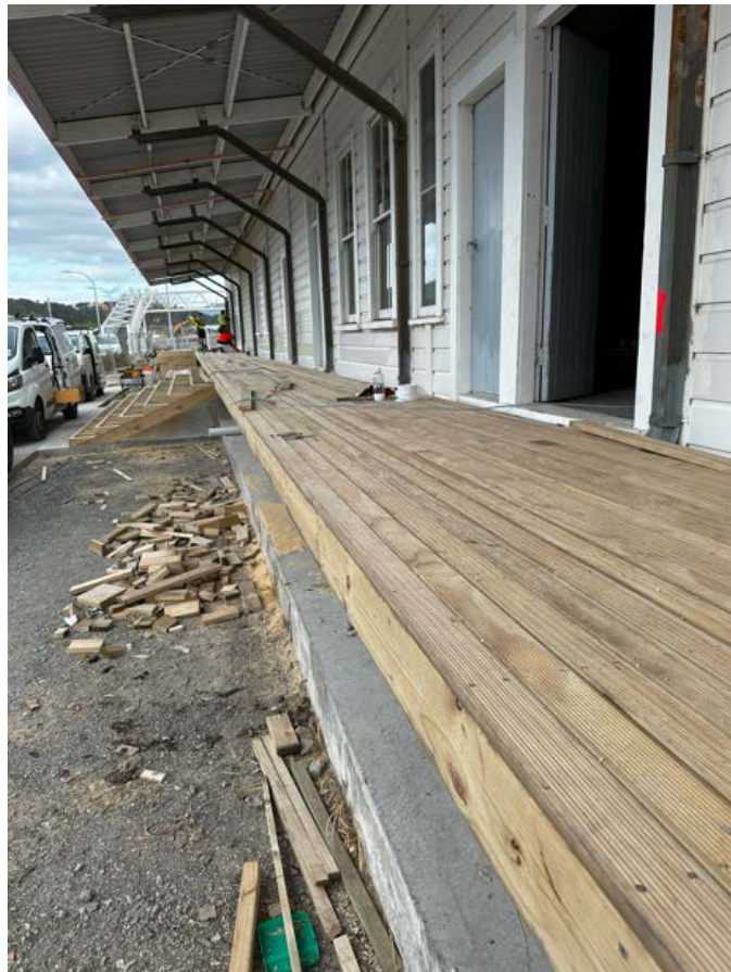
Decking being progressively completed
