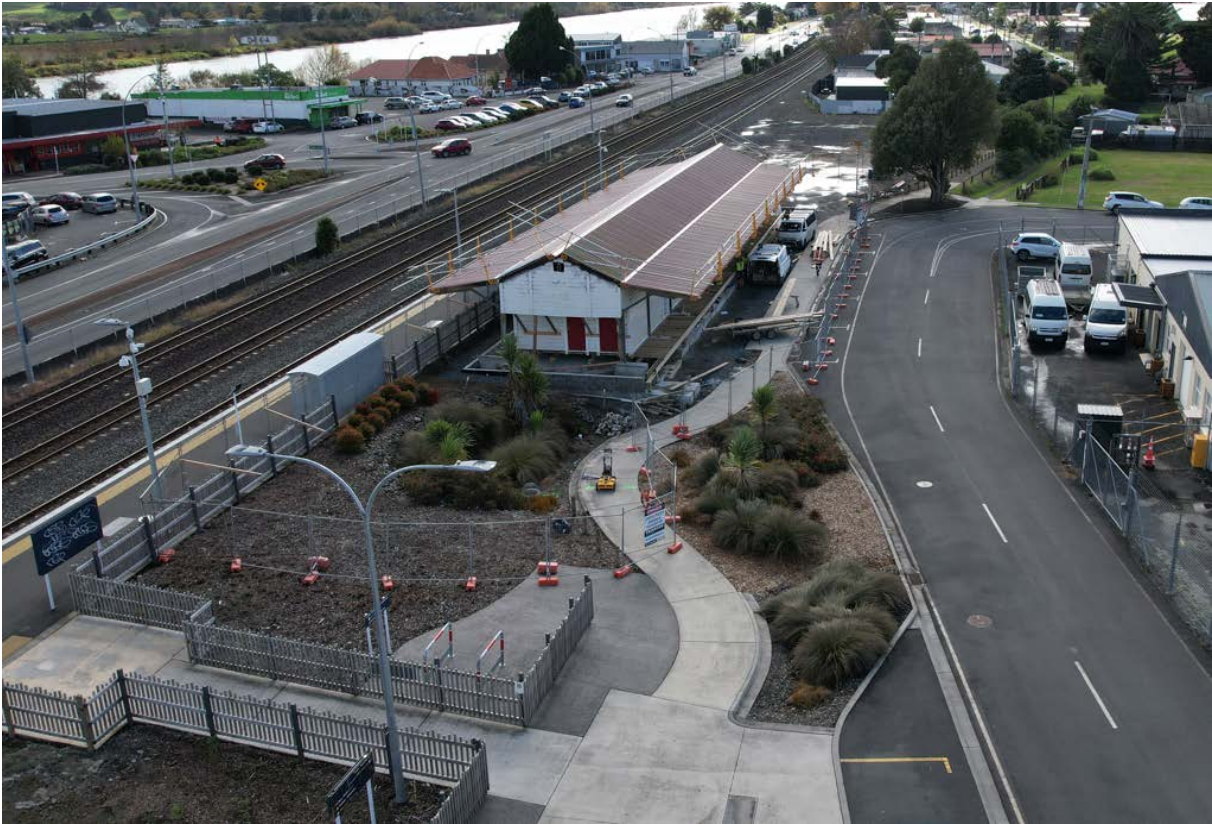
Roof replacement complete, with gutters yet to be completed
