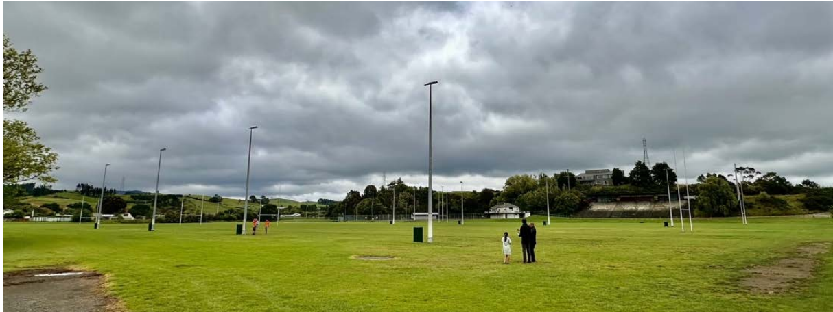
Completed lighting upgrade.
