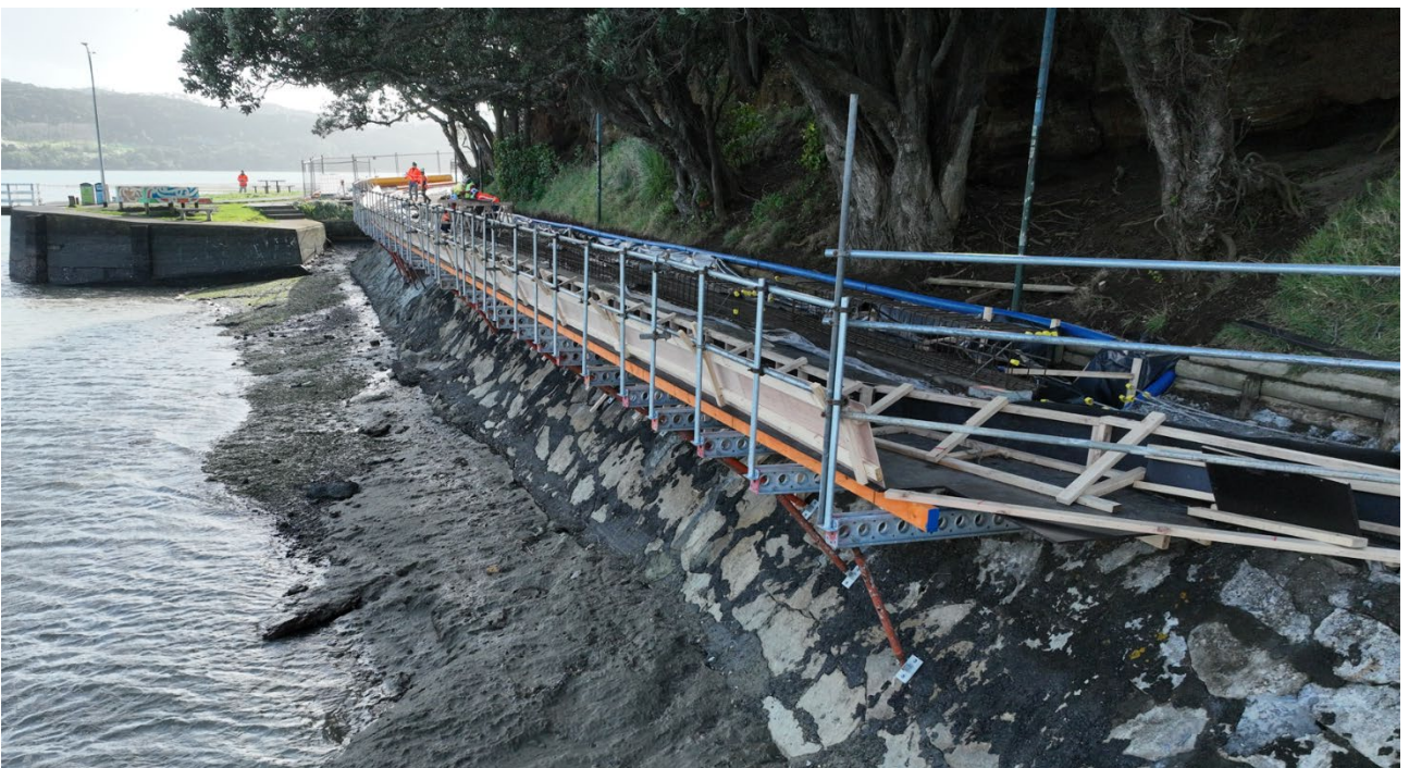
Temporary scaffolding to allow safe working
