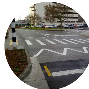
Raised pedestrian crossing
