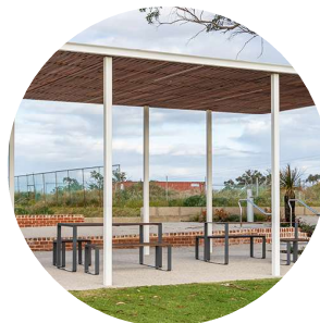
Shelter and shade at parks
